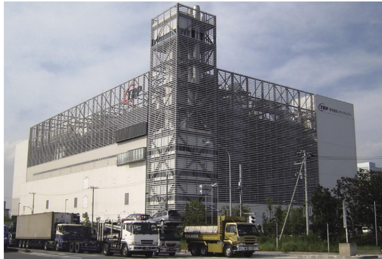
View of plant
