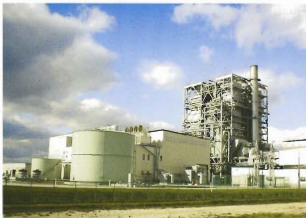
View of Tomakomai power plant
