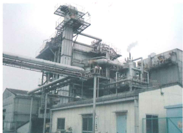
View of boiler at Ashikaga Plant
