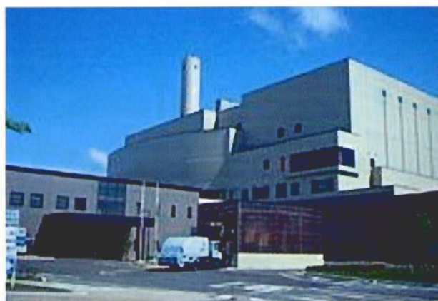
Sakata Area Waste Treatment Facility
