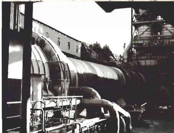
Giant rotary kiln (at the Tokuyama Factory)
