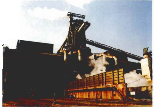
Plastic waste in powdered form is injected through the tuyeres near the bottom of blast furnaces to act as a reducing agent during the ore reduction and smelting process.
