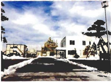
Shown here is the front entrance to the Niigata Plastic Liquefaction Center. The building on the right is for offices and the liquefaction plant can be seen in the background.
