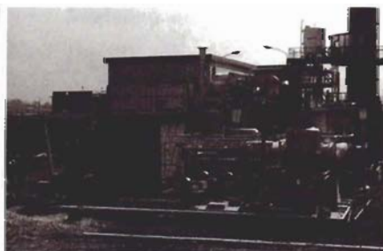
Facility in Koshigaya City for the experimental and specialized incineration of municipal plastic waste from sorted collections
