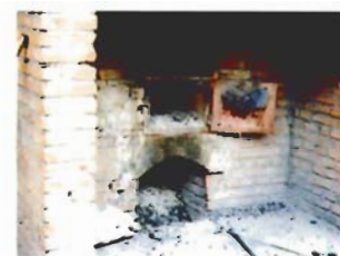
Heating by coal
