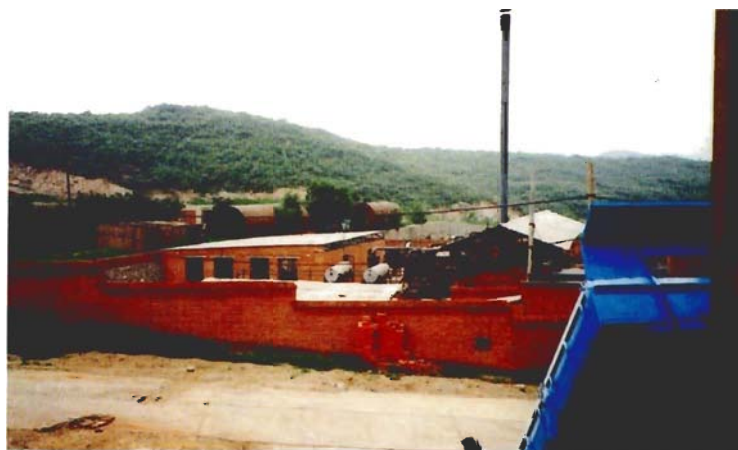
Overview of pyrolysis plant
